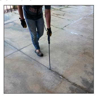
3. Once both the ACR Crack & Void and ACR Accelerating Agent have been applied. Allow the application to dry to the touch. Once dry to the touch, begin washing the excess material from the surface of the concrete.
