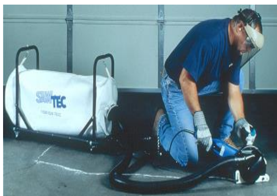
Photo #13 - Diamond Grinding
