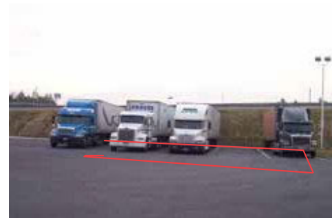
R-Tank HD Located Under Truck Parking Area
