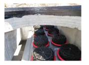
With the StormSafe chambers and new cartridges installed the maintenance process is complete. Re-install the manhole access covers and demobilize.
