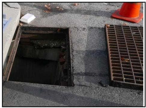
**2.** Measure and note the catch basin frame clear opening length and width. Remove any obstructions or debris that will interfere with the installed StormSack-BMP.
