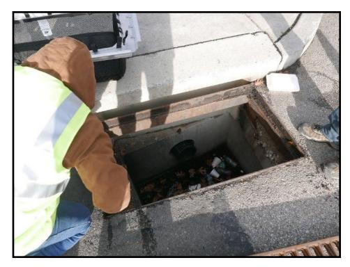
**3.** Prior to installing the StormSack BMP assembly, verify that the sack is secured to the support frame with the (6) locking rods. If not, simply insert StormSack tabs through the support frame slots, then secure the StormSack using the Locking Rods as shown (Geotextile Bags may vary from drawing).
