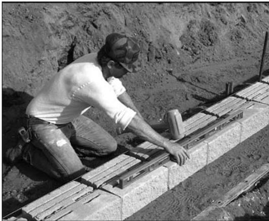
Align units using their backs or slots rather than their irregularly textured front faces. Stringlines may be helpful when aligning straight walls. Refer to pages 25, 26 and 27 for tips on curve and corner alignment. Place units side by side on the leveling pad. Front faces of adjacent units should fit tightly and unit bottoms should contact the leveling pad completely.
