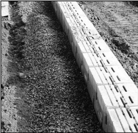
For walls over 3 feet high, perforated drain pipes should be used to collect water along the base of the drainage aggregate. Drain pipes help to quickly remove large amounts of water. For some projects, often shoreline applications, a geosynthetic filter fabric may be required behind the drainage aggregate. Filter fabric will prevent soils or sands (fines) from migrating into the drainage aggregate and wall face joints.
