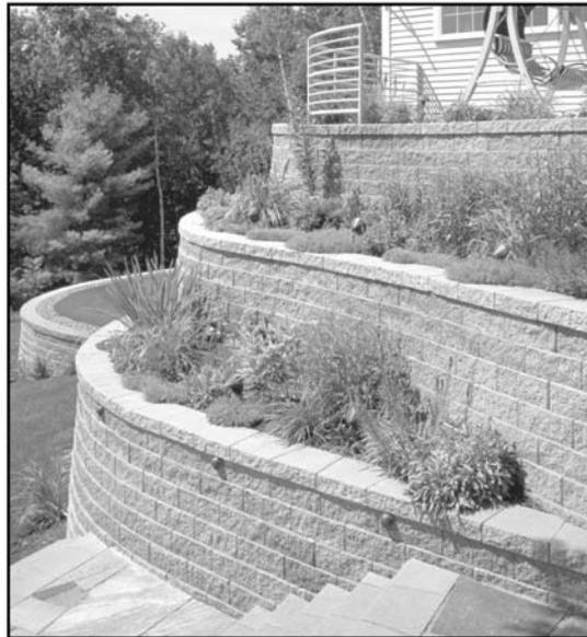
*Several closely spaced tiered walls can create steep, unstable slopes. If tiered walls make a grade change steeper than 2:1 (horizontal: vertical), global slope stability may need to be reviewed by a qualified soils engineer.*
