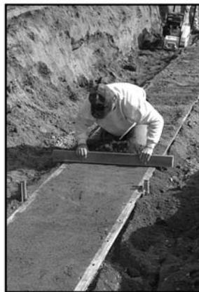
*To quickly construct long sections of leveling pad, create forms by leveling and staking rectangular metal tubing along both sides of the planned pad. Place and compact granular material within these leveled forms and screed off excess.*
