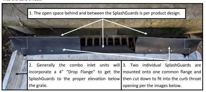
The image and notes above reinforce the basic look and concept of the dual SplashGuard flange associated with ScreenBox installations in combination (curb throat) inlets.
