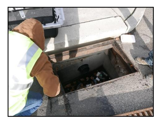
**3.** Using the catch basin frame clear opening length and width measurements from Step 2, adjust the sliding flanges such that they will securely rest on the grate frame. The inside flange to flange distance should be equal to the previously measured clear space for both length and width.
