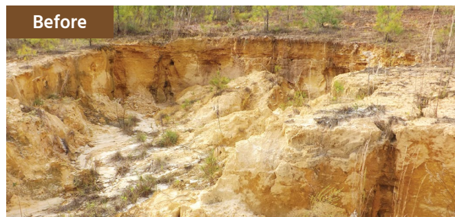
Large gullies formed due to erosion
