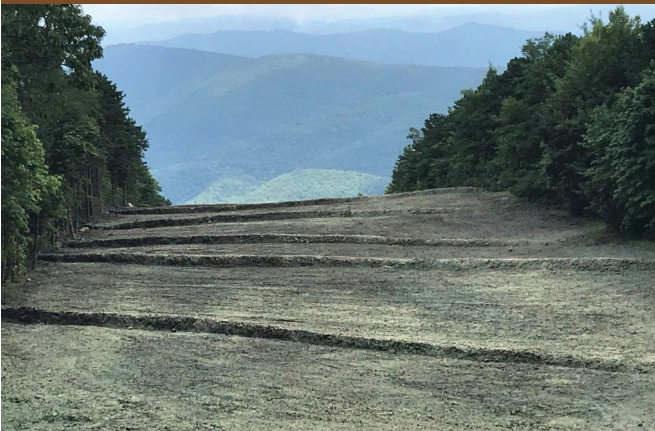
Energy / Pipeline Restoration
