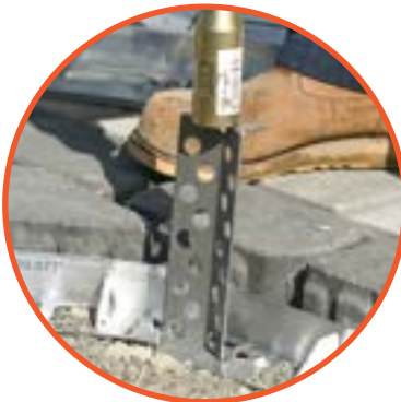
PERMEABLE (OPEN GRADE) BASE SOLUTION Install QUICK-E-Hybrid Stake
