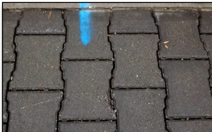
Photo 2 – PaveDrain following maintenance
