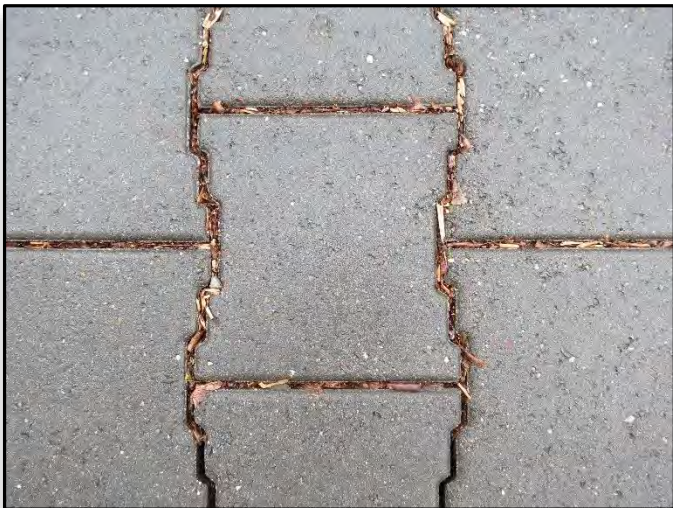
Just one pass of an Elgin Whirlwind Vacuum Truck over the PaveDrain System filled with mulch and road debris.
