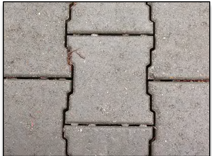
Just one pass of an Elgin Whirlwind Vacuum Truck over the PaveDrain System filled with mulch and road debris.
