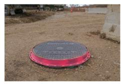
**STEP 6:** The drain basin body can be cut at the time of the final grade or raised with riser. No brick, stone or concrete block will be required to set the grate to the final grade height.
