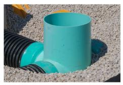
**STEP 5:** Backfill uniformly around structures with class I, II, or III material and compact in lifts according to ASTM D2321.
