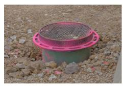
**NOTE:** For H-20 or heavier load rated installations, set elevation of frame and grate. Then pour a concrete collar around and knife flowable fill under edges to support the frame.
