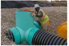
**STEP 4:** Backfill the back side of structures and push the pipe home to the seat position. Re-check Drain Basin depth, level and position.
