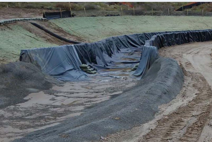
MW used as a diversion channel
