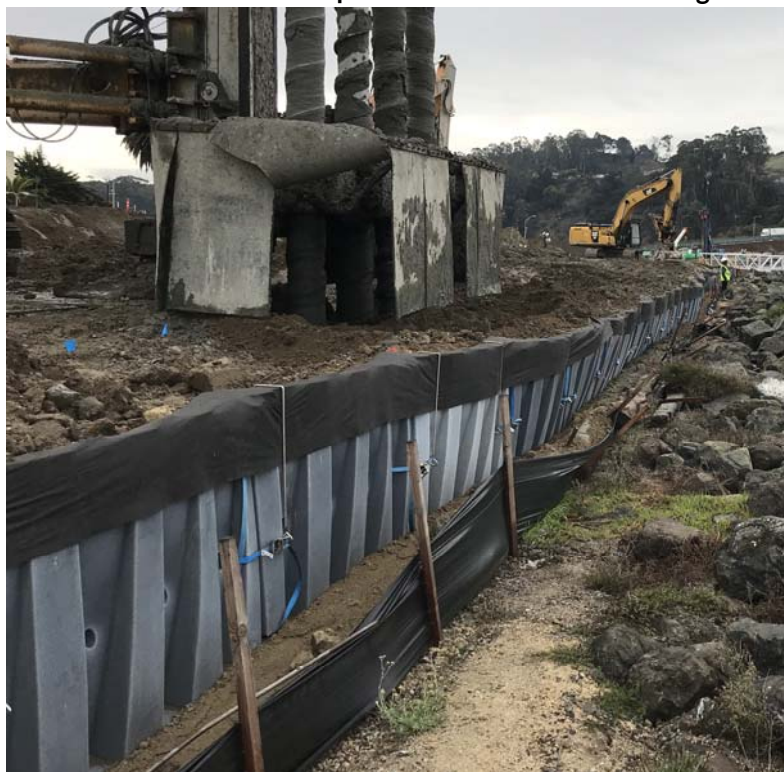
MW used as a robust perimeter control and retaining wall
