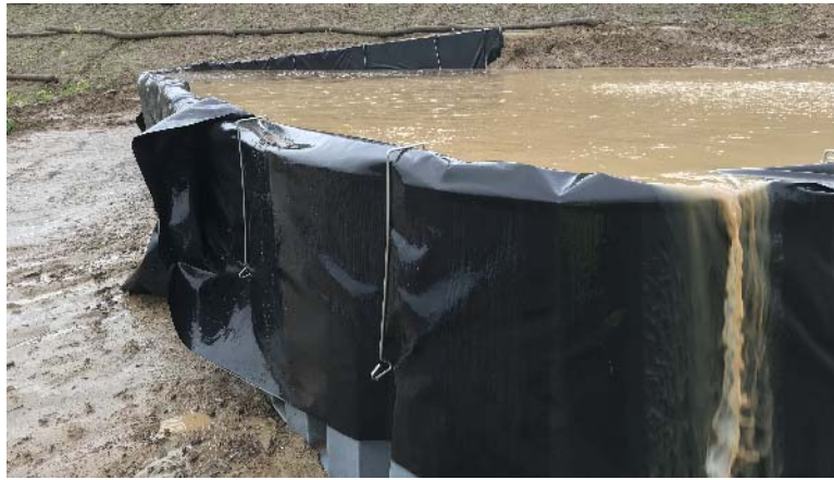
Figure 12: Basin MW-9 overtopping during a storm event.
