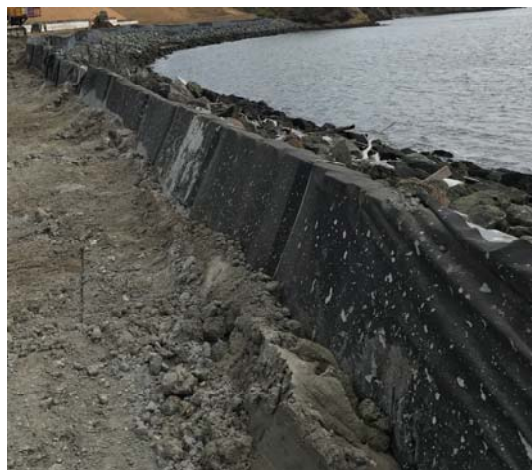
Muscle Wall as a liquid waste containment barrier
