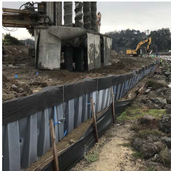
Muscle Wall as a temporary retaining wall for soil
