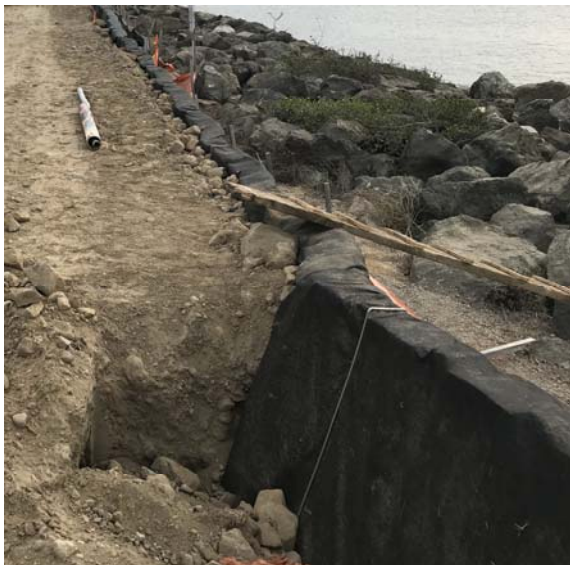
Muscle Wall as a temporary retaining wall for soil
