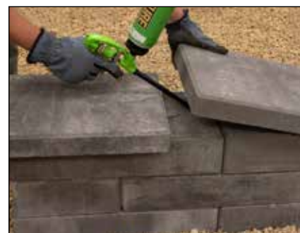
Diagram 3—Capping the Wall
