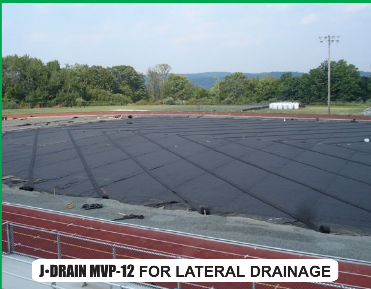
DRAINAGE LATERALS INTO SIDELINE TRENCH
