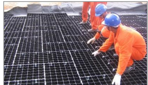
Figure 15: Connecting GEOTERRA Units
