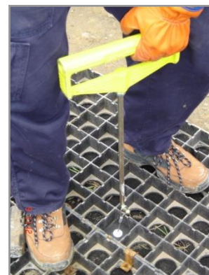
Figure 33: Setting the Earth Anchor
