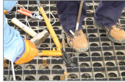
Figure 34: Crimping the Cable Stop
