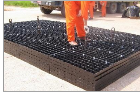
Figure 28: Assembling GEOTERRA Mats (Side-by-Side Pattern)
