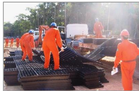
Figure 26: Transporting Pre-Assembled Mats from Off-Site
