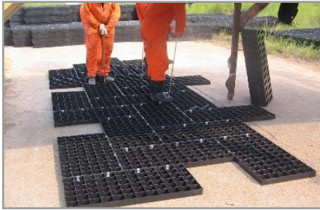
Figure 27: Assembling GEOTERRA Mats (Herringbone Pattern)
