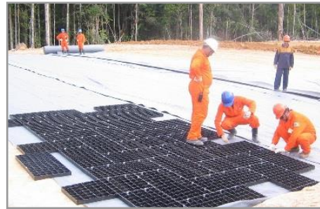
Figure 29: Placing GEOTERRA Mats Over Geotextile Layer
