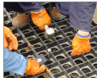
Figure 32: Driving the Anchor Head
