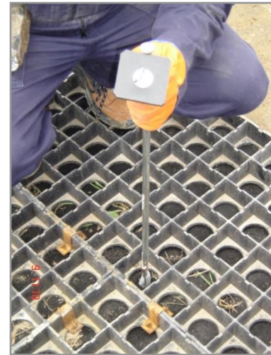
Figure 31: Installing the Earth Anchor
