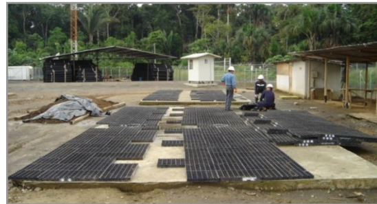
Figure 30: Connecting Pre-Assembled GEOTERRA Mats
