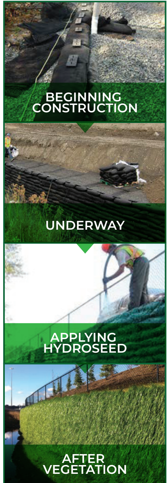
5m (16ft) tall commercial retaining wall
