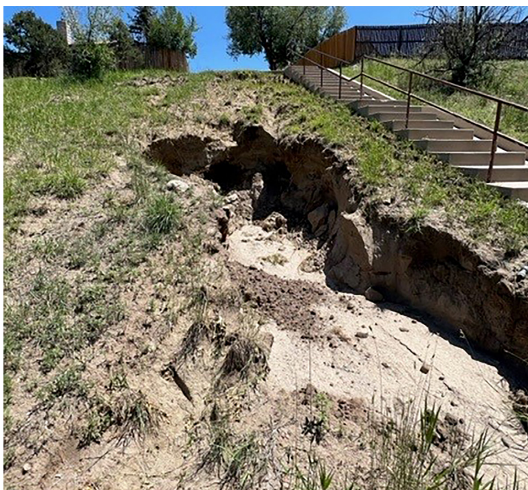
Pictures of the erosion problem before Concrete Canvas® installation.
