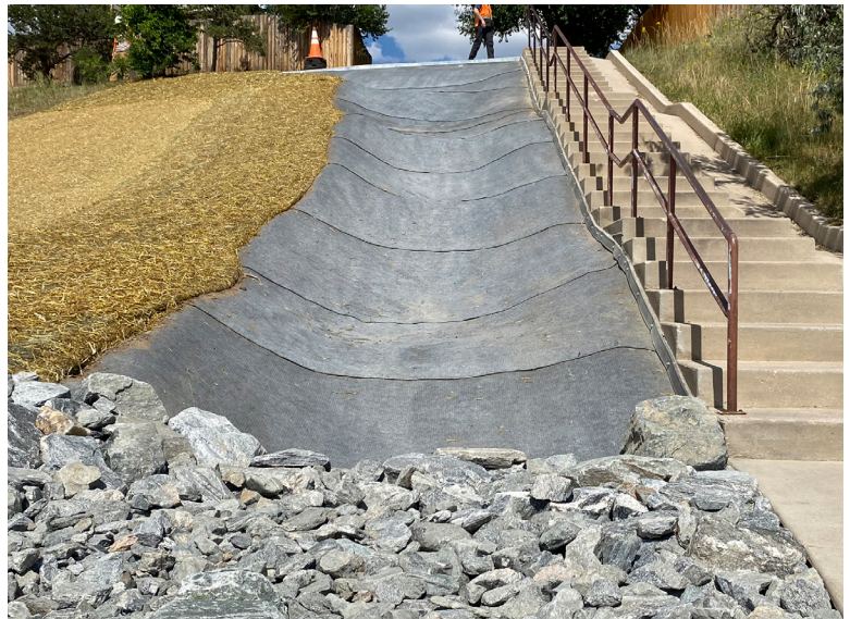
Concrete Canvas® Laid Transversely Across the Slope & Rolling Berms
