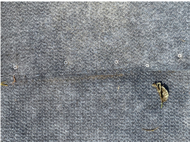
Overlapped CC Layers Secured Using Stainless Steel Screws
