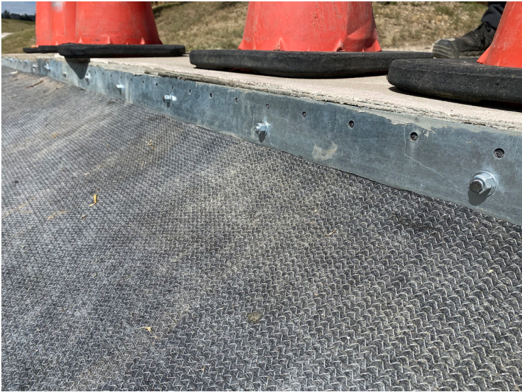
Concrete Canvas® Attached to Concrete with Stainless Steel Clamping Bar and Through-Bolts, a Gasket & a Grout Filler
