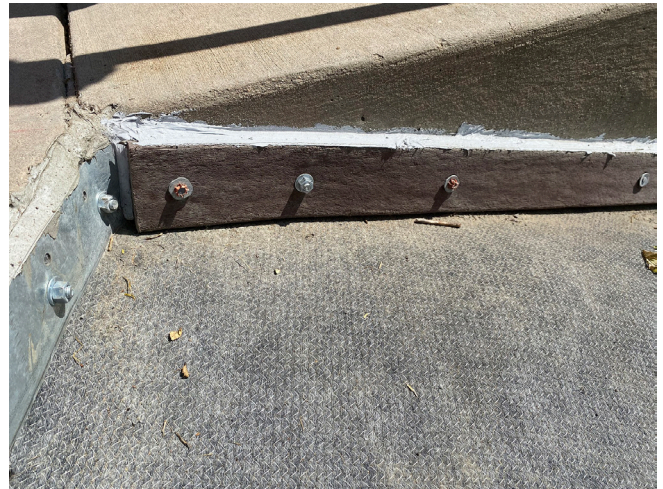
Concrete Canvas® Attached to Concrete with Stainless Steel Clamping Bar and Through-Bolts, a Gasket & a Grout Filler
