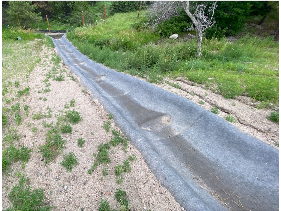
Completed Concrete Canvas® Installation
