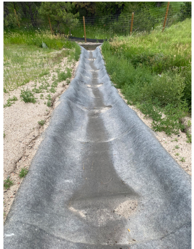
Completed Concrete Canvas® Installation
