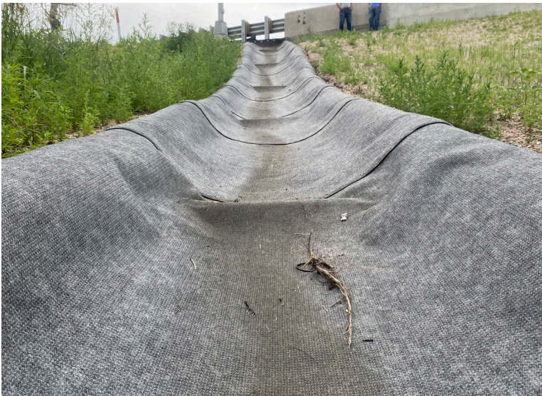
Concrete Canvas® Laid Transversely Across the Channel
