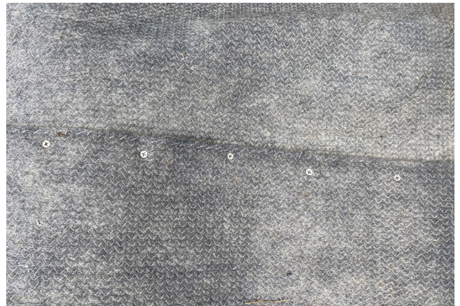
Overlapped CC Layers Secured Using Stainless Steel Screws
