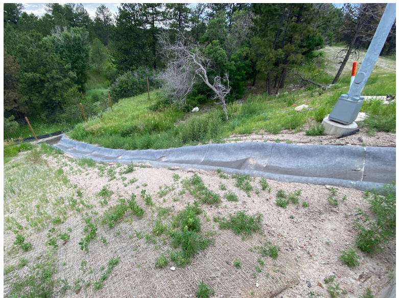
Completed Concrete Canvas® Installation
