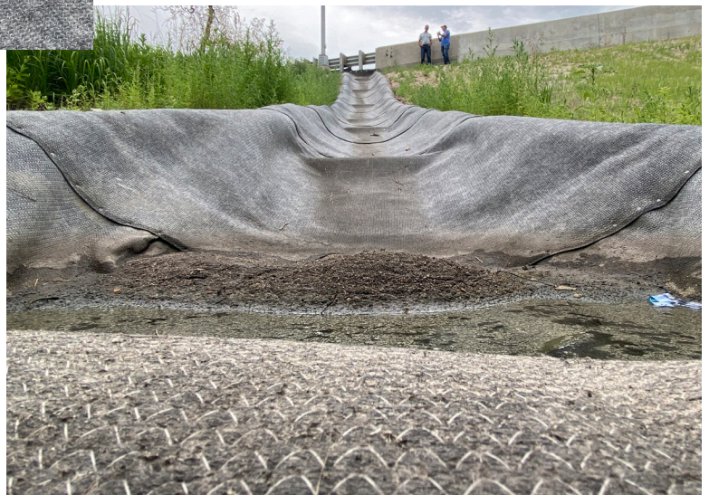
Check Dams & Dissipation Pond Covered in Concrete Canvas®
