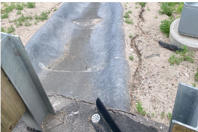
Concrete Canvas® Secured with Anchor Trenches
