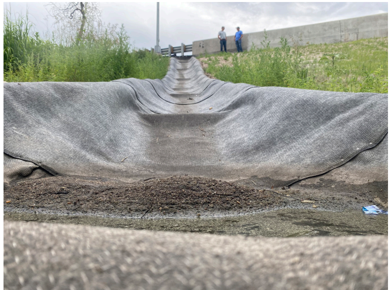
Completed Concrete Canvas® Installation
