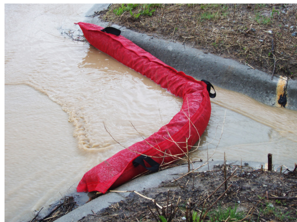
Big Red CI protector protecting a concrete swale.
