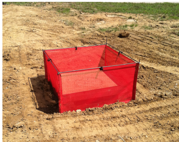
Big Red AI Protector, recently installed with trenched in bottom and tight sides.
