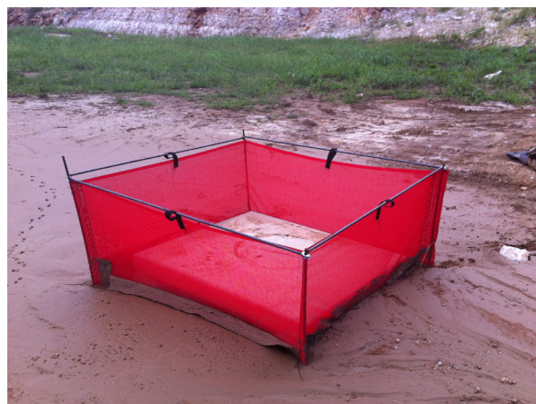
Big Red AI Protector with 4" sediment load after initial rain event.
