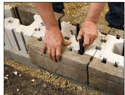
Diagram 20—Placing veneers onto modular block
