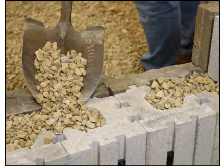
Diagram 5—Fill cores with free draining aggregate
