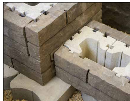
Diagram 23—Ending a wall at a column example
