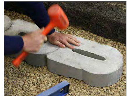
Diagram 19—Lay and level base block
