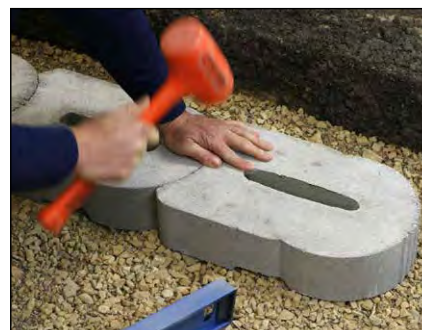
Diagram 3—Lay and level base block
