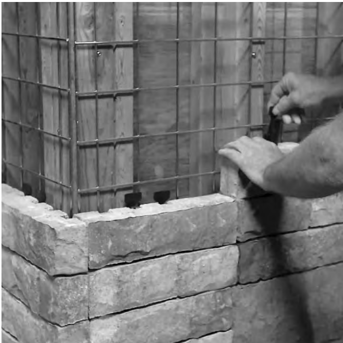
Attach Lafitt Tandem Veneer with Connector
