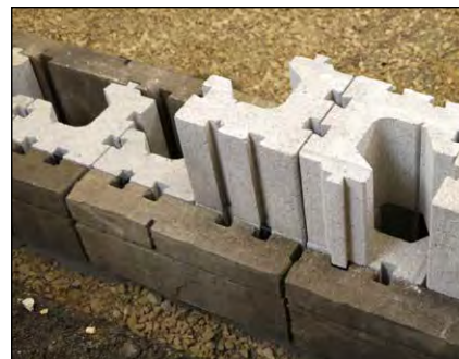
Diagram 21—Second course construction
