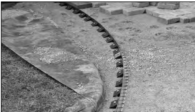
Install edge restraints.
