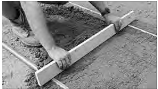
Install bedding sand.
