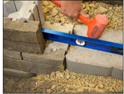
Diagram 7—Stepping up the base
