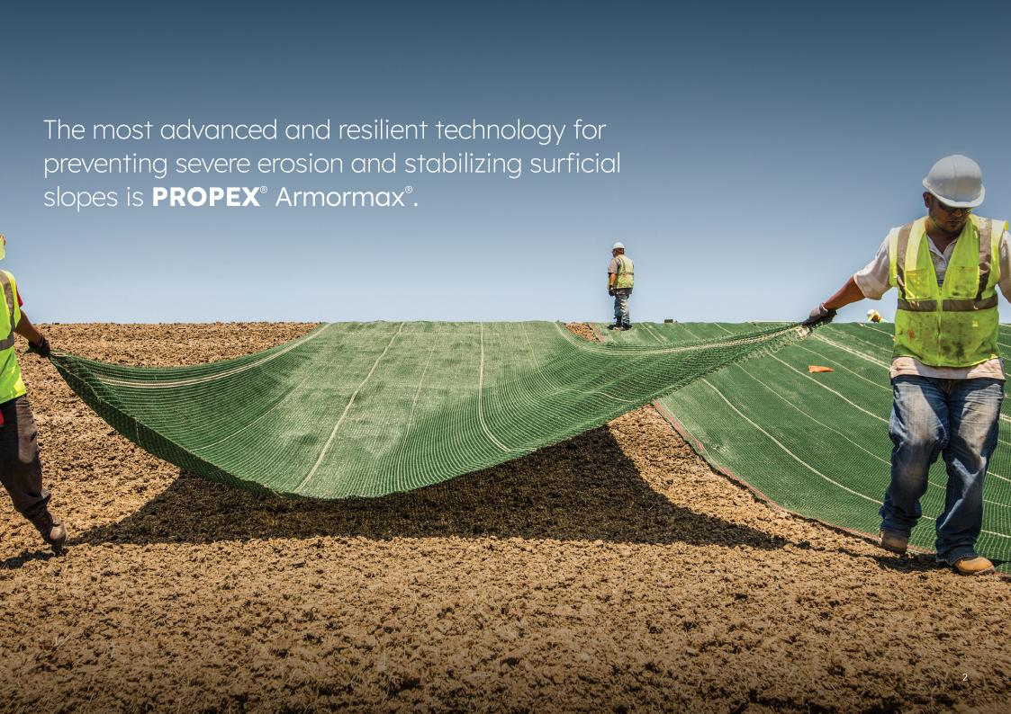
PROPEX Armormax is composed of High Performance Turf Reinforcement Mat (HPTRM) and Engineered Earth Anchors that work together to lock soil in place and protect against hydraulic stresses.
