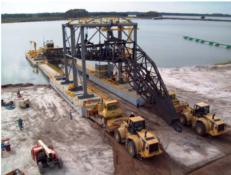
Figure 11. Final push during launching.
