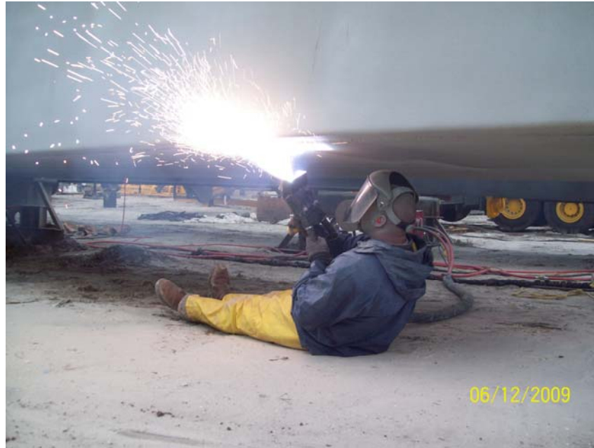
Figure 9. Thermal arc spray application.
